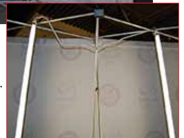
Link cable connection close up.
